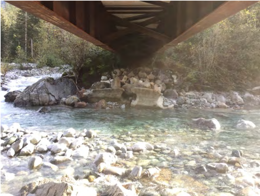
Left Bank Abutment when facing downstream
