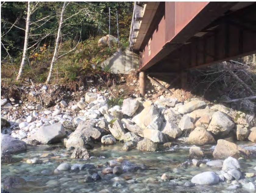
Fill at right bank is over steepened
