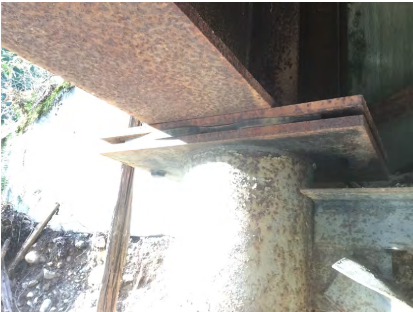
Bearing pads at right bank
