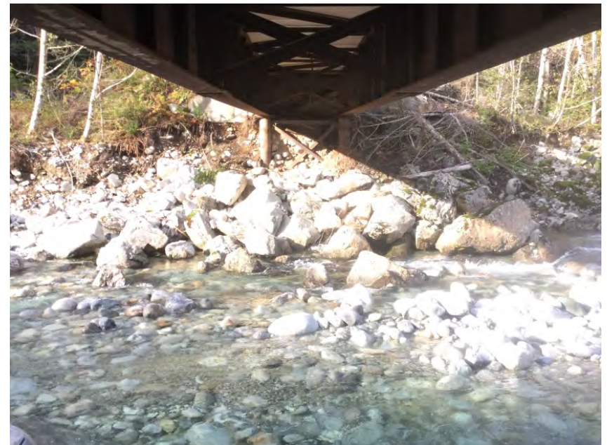
Right Bank Abutment when facing downstream
